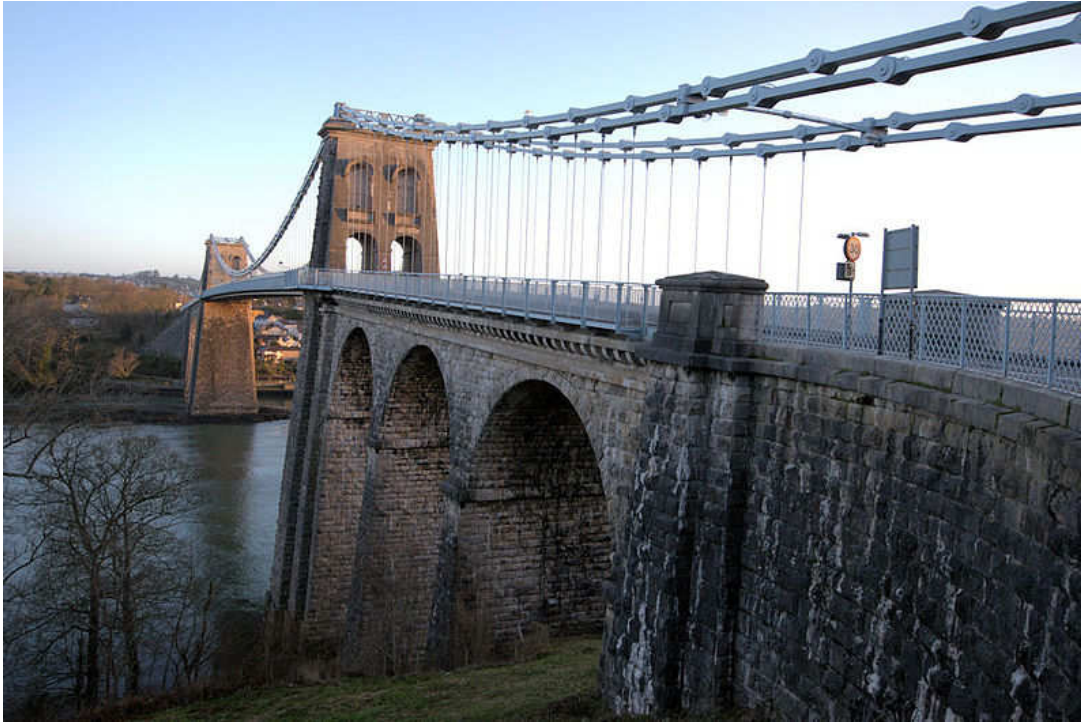
Menai Suspension Bridge
